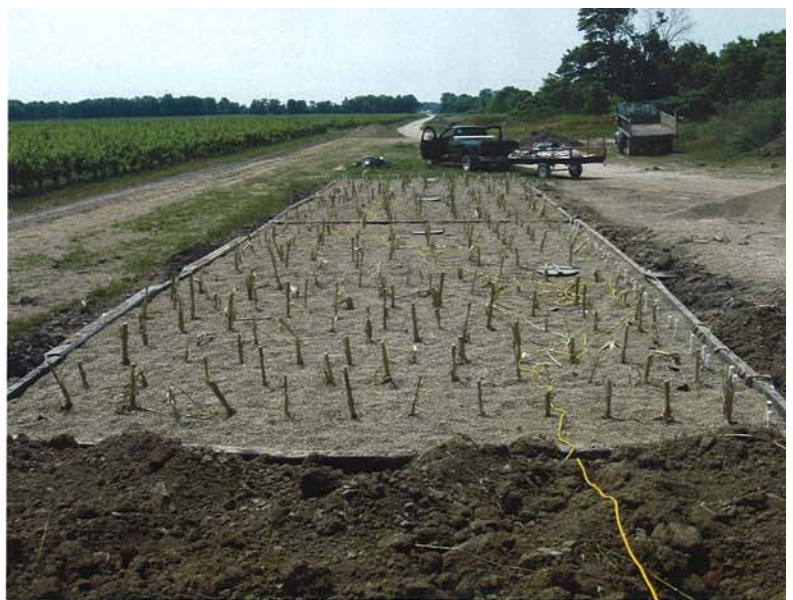
Newly completed Wetland Biofilter System.
